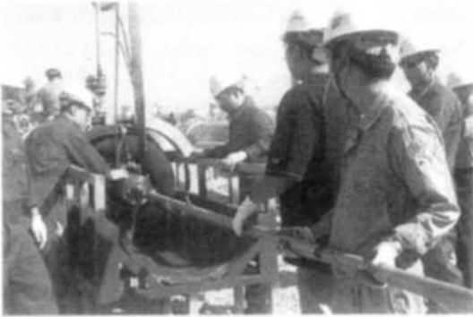
Fig. 14 Injecting the PIG into the pipeline
